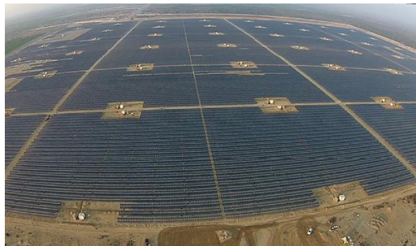
Figure 2: Drone camera image of the Pakistan's first, and the world's largest, grid-connected solar power plant (100 MW), inaugurated on 5th May 2015.
